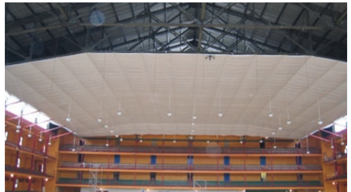
Dropped below structural steel — installation shown in progress
