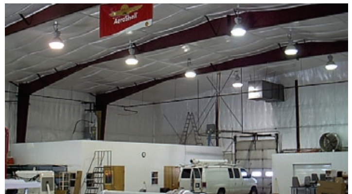
Energy Miser® installed under purlins
