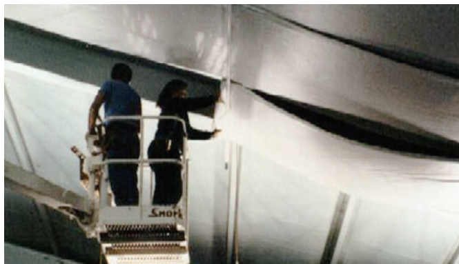
Installation of the Energy Miser® system
