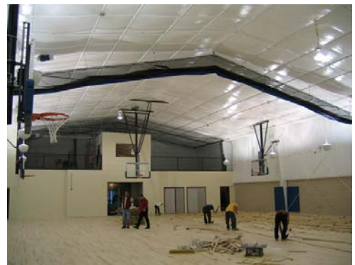
Flooring Installation Nov. 2003
