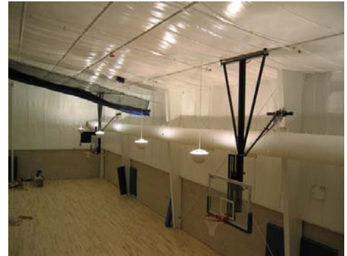
Interior Finish Nov. 2003
